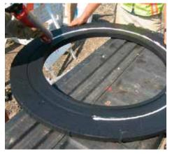
For Angle Rings, place a 1/4" bead of M-1 into the groove on the underside of the Angle Ring and to the inside shoulder of the Finish Ring.
