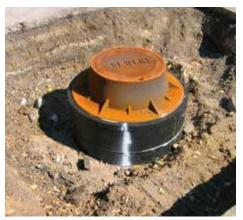
If Angle Rings are used, a paint mark should be made on the rings during dry fit alignment to ensure proper position once installed with the adhesive. Once final elevation is set, remove the ring stack and set upside down off to the side.
