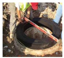
Embed the first ring directly into the mortar, center it and make sure the ring is level. Proceed to step 6 to determine remaining rings required. If step 3&4 are not required, proceed to step 5.
